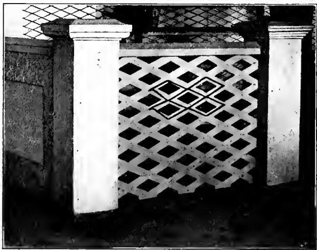
Fig. 124 —Lattice Design of Panel
